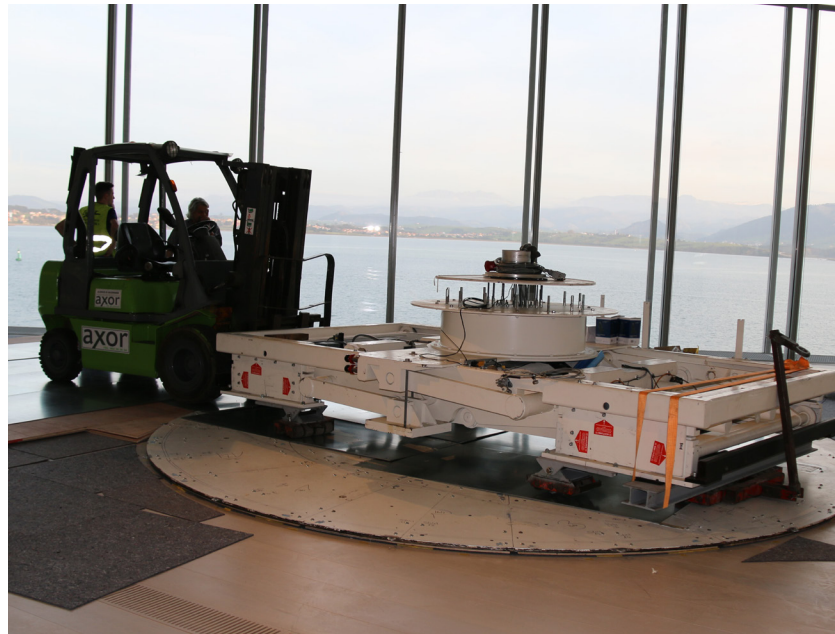
POSITIONING THE LIFT ON THE BASEPLATES
