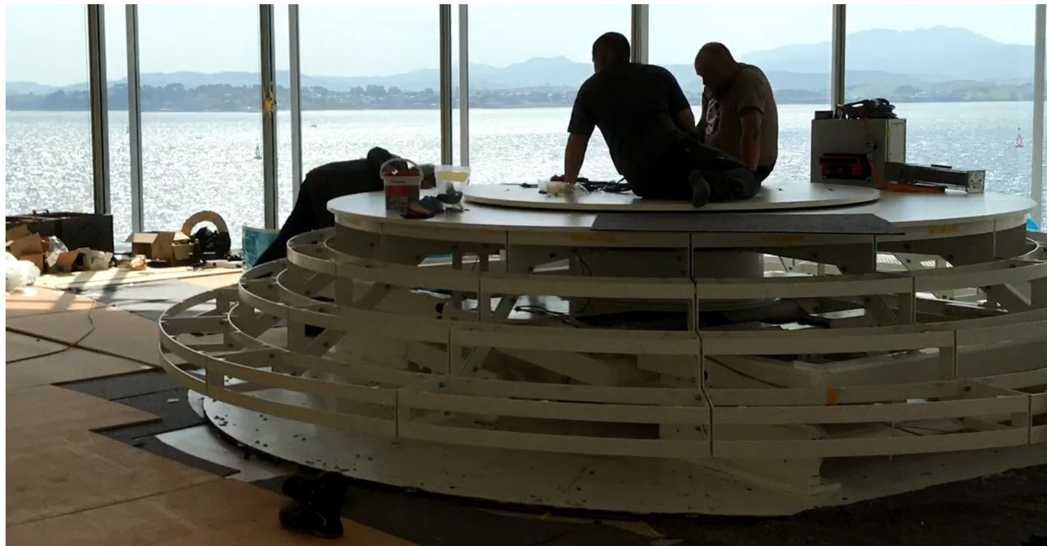
INSTALLING THE TURNTABLE
