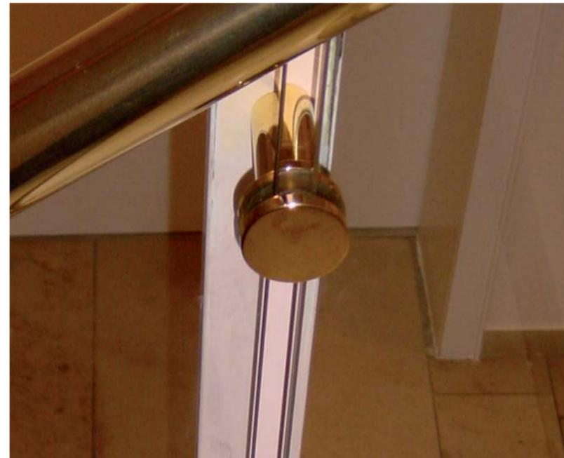
VERGOLDETES HALTEELEMENT KLEMMT DIE GLASSCHEIBEN AUS ESG 10MM KLARGLAS.
