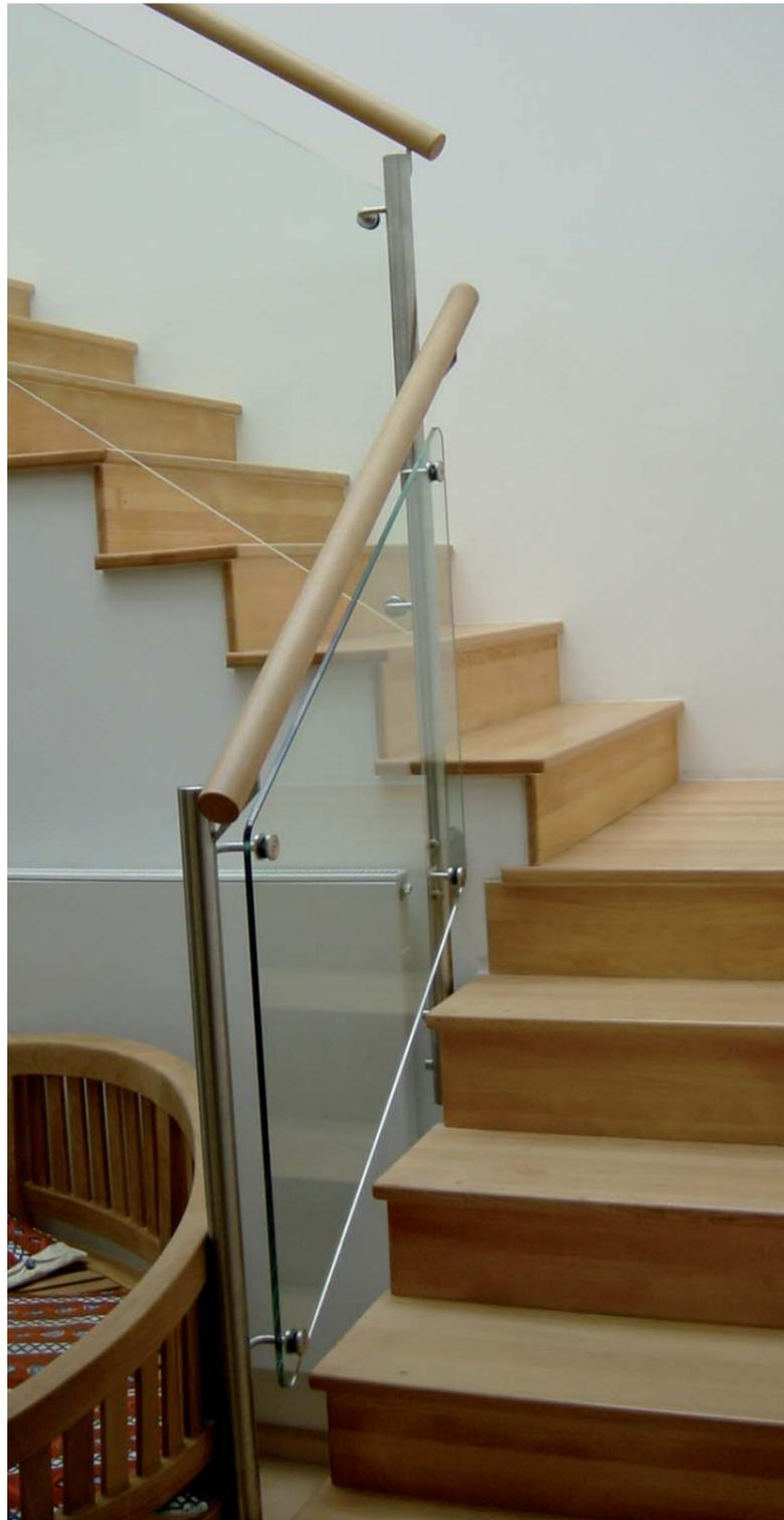
VERSCHRAUBTE GLASELEMENTE AN EDELSTAHLPFOSTEN MIT HOLZHANDLÄUFEN
